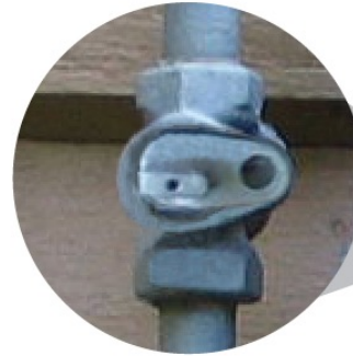
Closed gas meter valve
